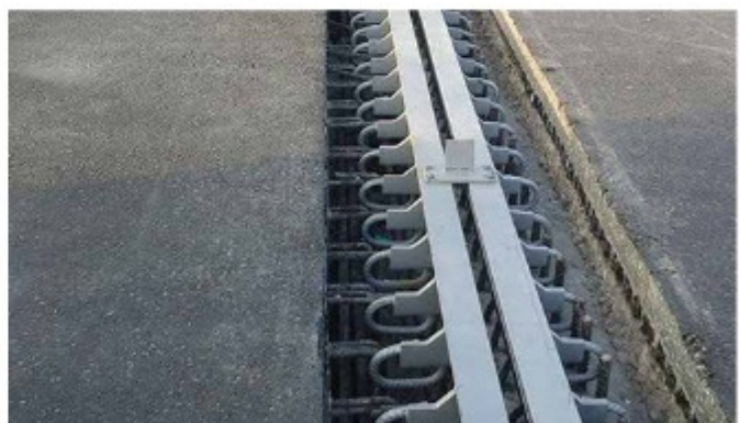
Installation of AR-EX HS
