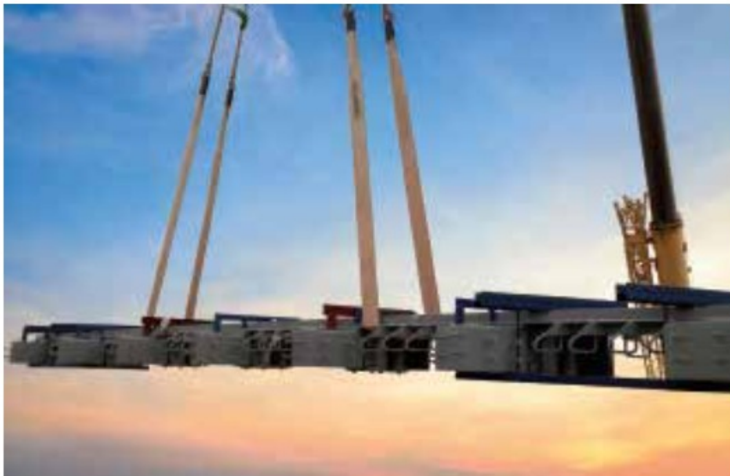
Installation of AR-EX Expansion Joints
