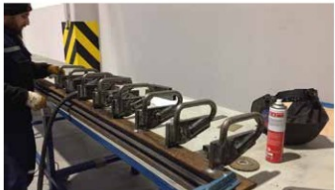
Anchorage Welding of AR-EX HS
